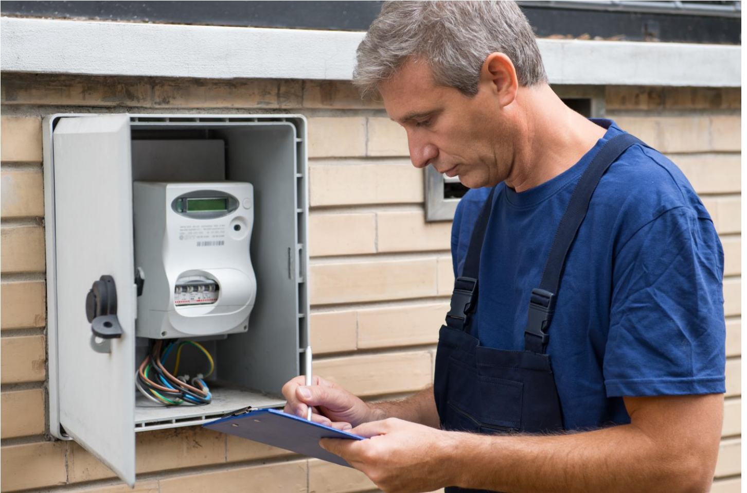
Utility employee setting up new utilities for a relocation client.
